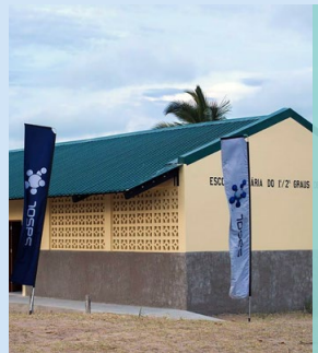
Rehabilitated classrooms – Inhassoro
